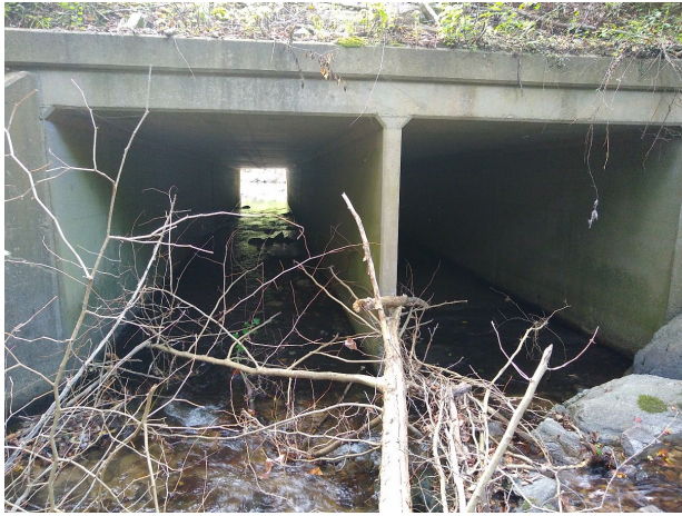
Eastbound exit ramp culverts in Cold Springs - downstream view.
