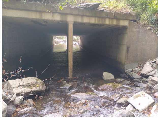
Westbound entrance ramp culverts in Cold Springs - downstream view.
